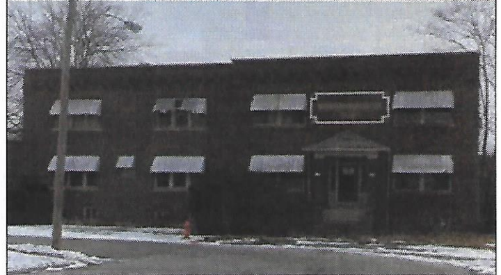
Top and center: Two historic views of the old Federal Paperboard Office at 960 East North Street. Photos provided by David Belden and the Local History Project digital collections. Bottom: The paper mill building today. Photo by your editor.
